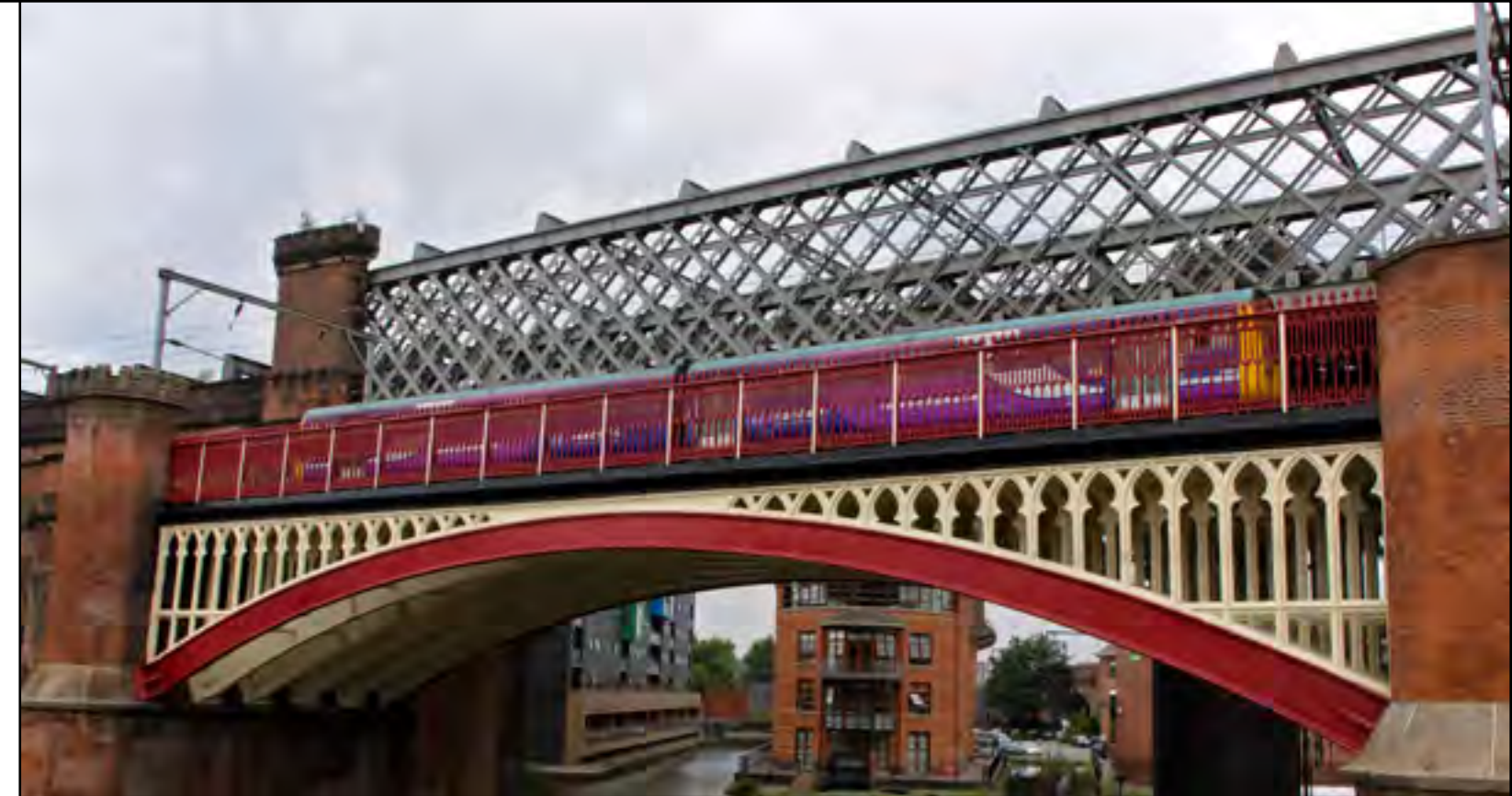
Above: A rather late running Class 142 crosses 'No.100A' the freshly painted 1849 South Junction and Altrincham Railway's cast iron arch bridge over the Rochdale Canal into Knott Mill railway station (Deansgate) on August 8th. Colin Irwin
