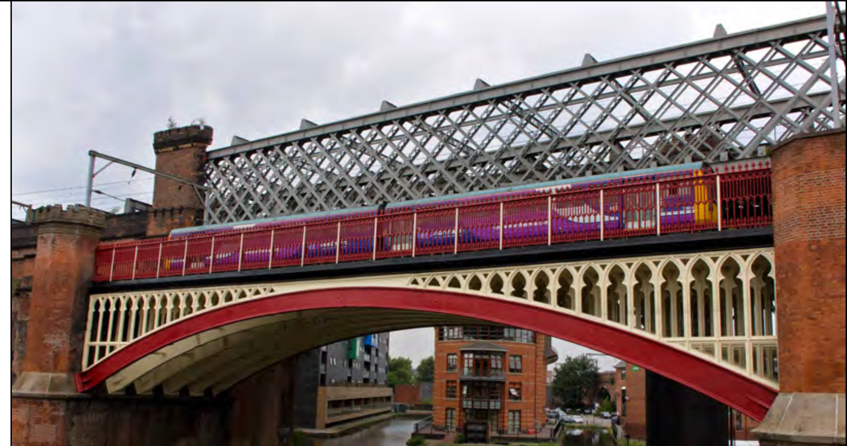
Above: A rather late running Class 142 crosses 'No.100A' the freshly painted 1849 South Junction and Altrincham Railway's cast iron arch bridge over the Rochdale Canal into Knott Mill railway station (Deansgate) on August 8th. Colin Irwin
