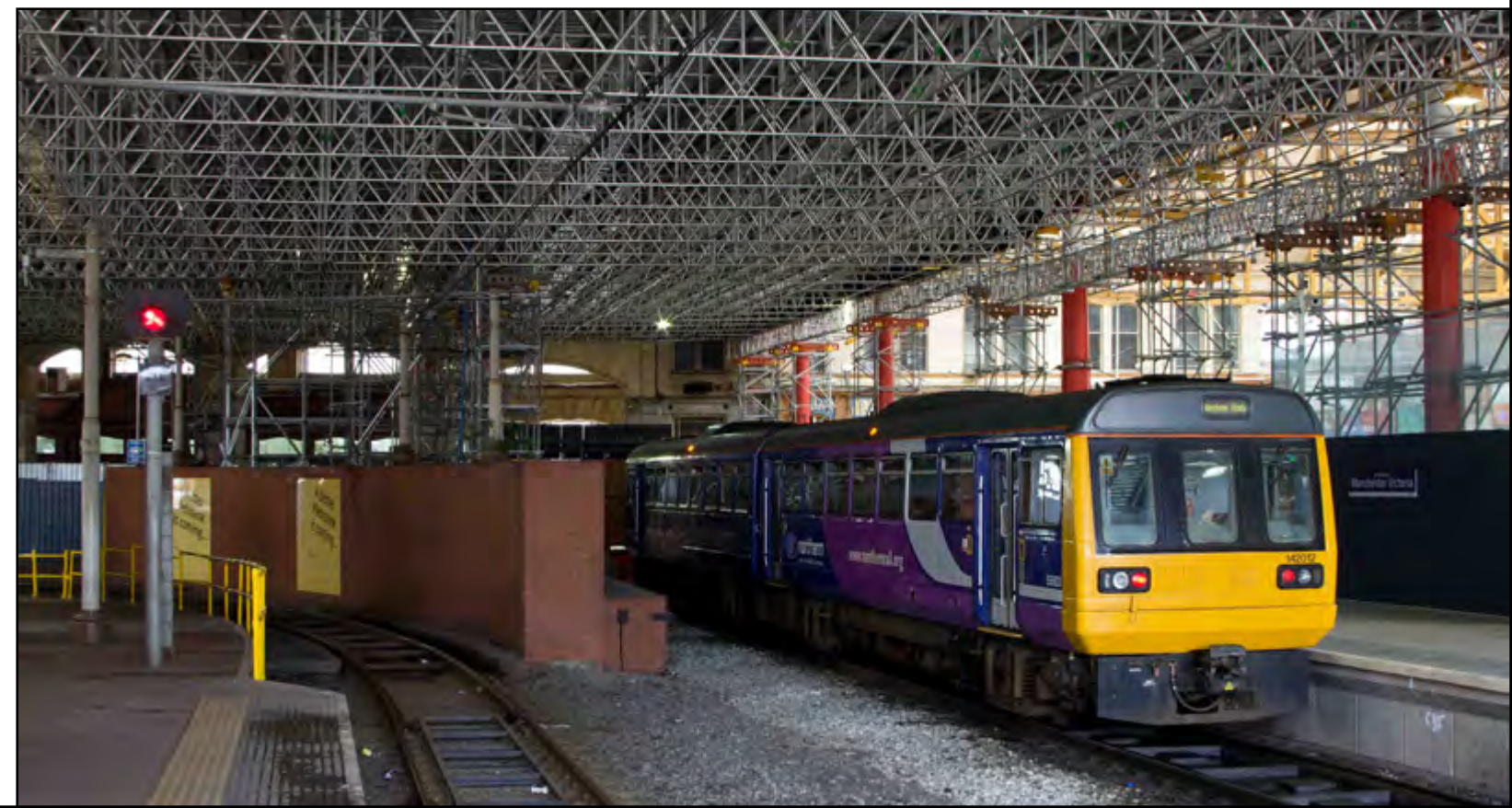
Below: On August 18th, Class 142 012 sits under Manchester Victoria's new roof of scaffolding, now that the original 1844 roof has been removed over platforms 1 & 2 in preparation for the new glass to be installed. Colin Irwin
