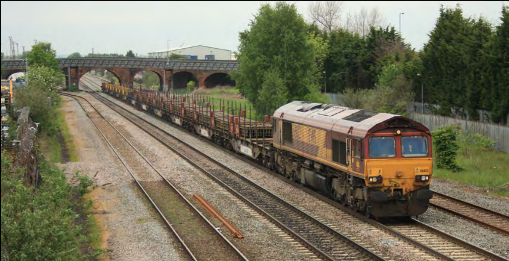
Above: Class 66 012 with 6X01 Scunthorpe - Eastleigh hauling new continuous welded rail heads through Burton on Trent, May 21st. Stuart Hillis
