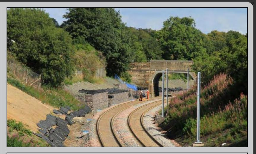
Above: With the trackwork almost complete the embankments get tidied up and drainage installed. *Jonathan McGurk*Below: The stantions are in place for the electrification team to start the task of wiring the route. *Jonathan McGurk*
