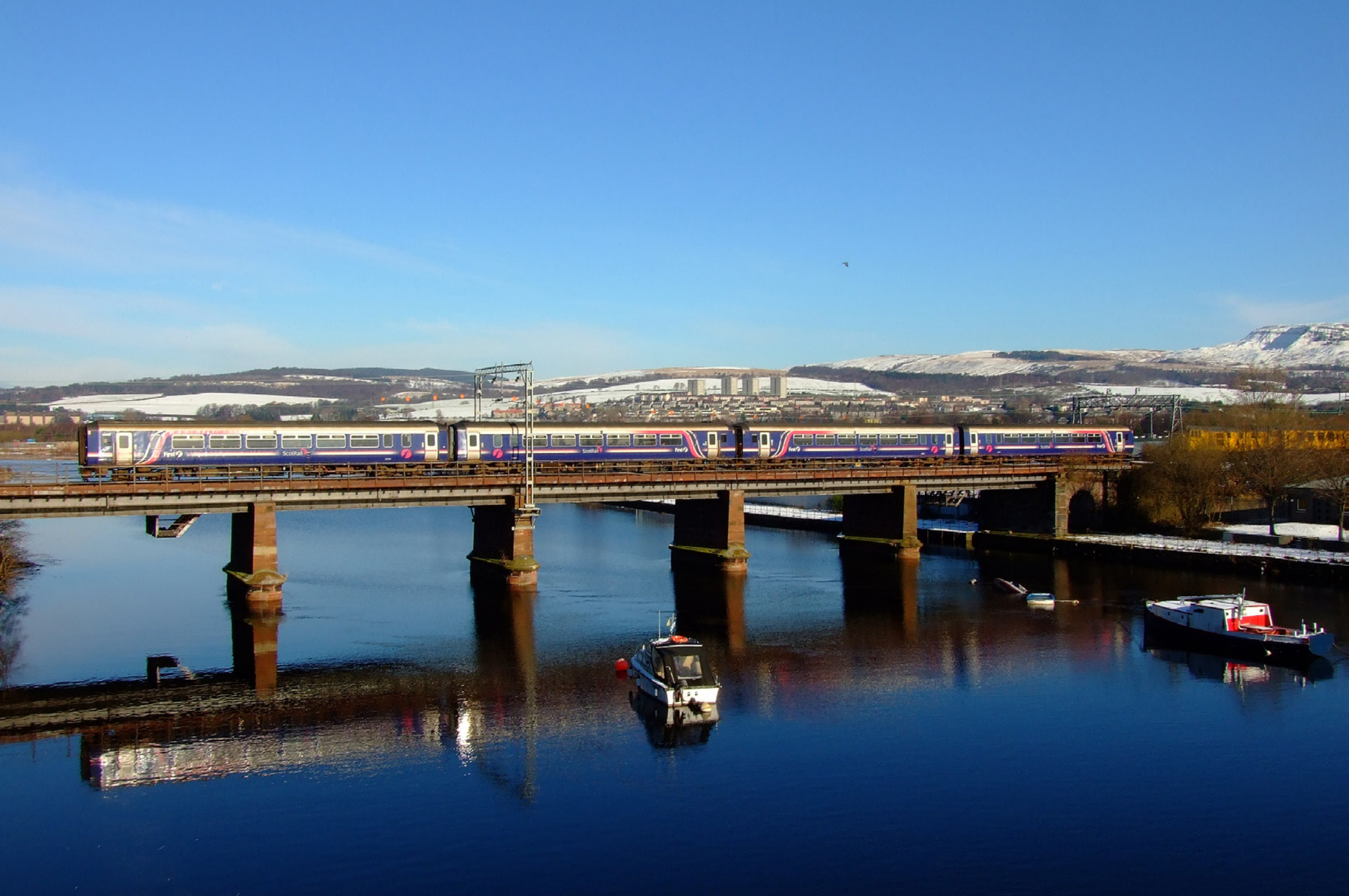
Reflecting on the River Leven, Class 156 493 is seen leading a four car train which is seen crossing over Dalreoch Viaduct heading towards Helensburgh Upper on the 10th February. Jonathan McGurk
