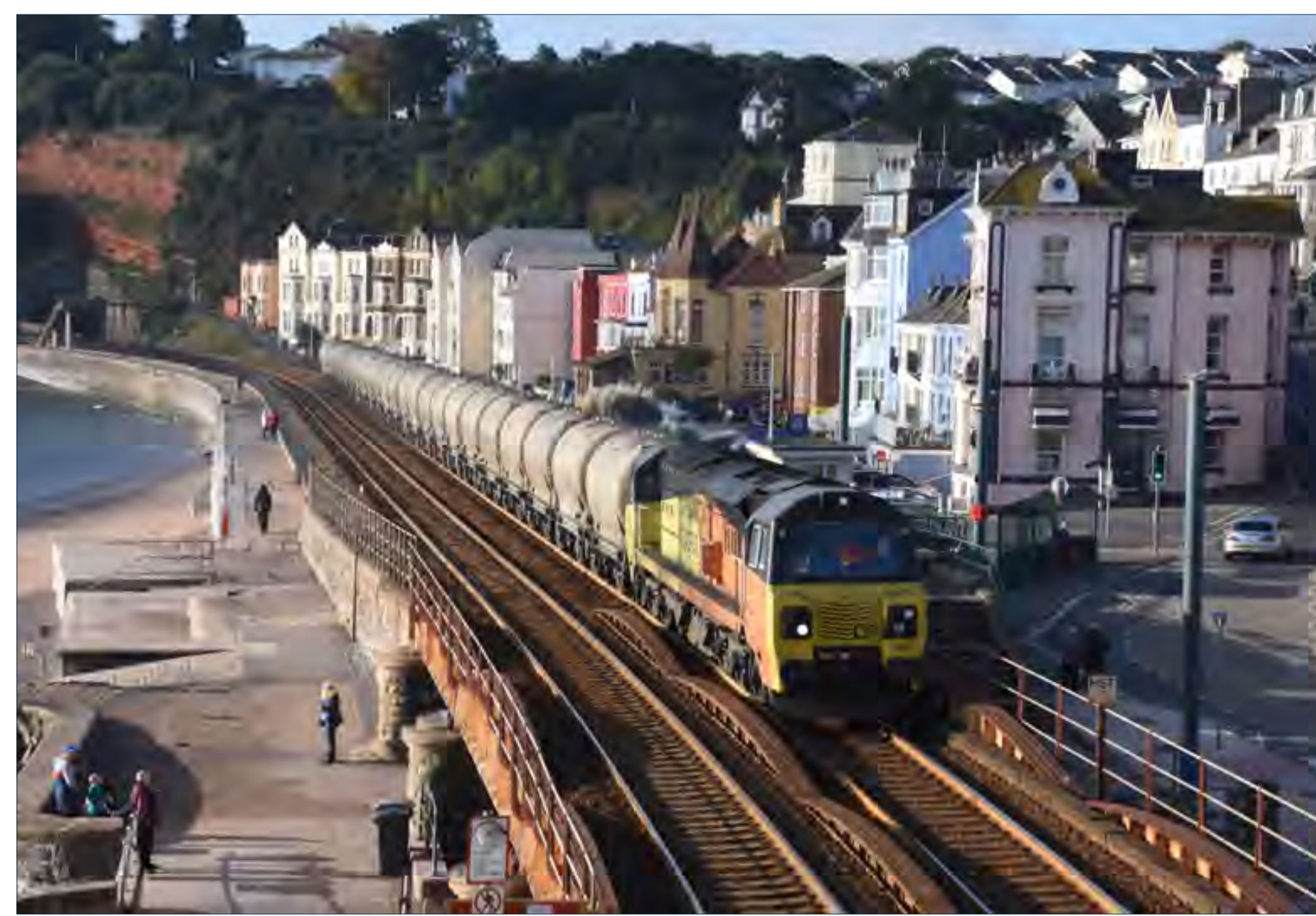
On October 25th, Class 70 807 hauls the 6C36 Moorswater - Aberthaw comprising 23 empty PCAs through Dawlish. Steve Thompson
