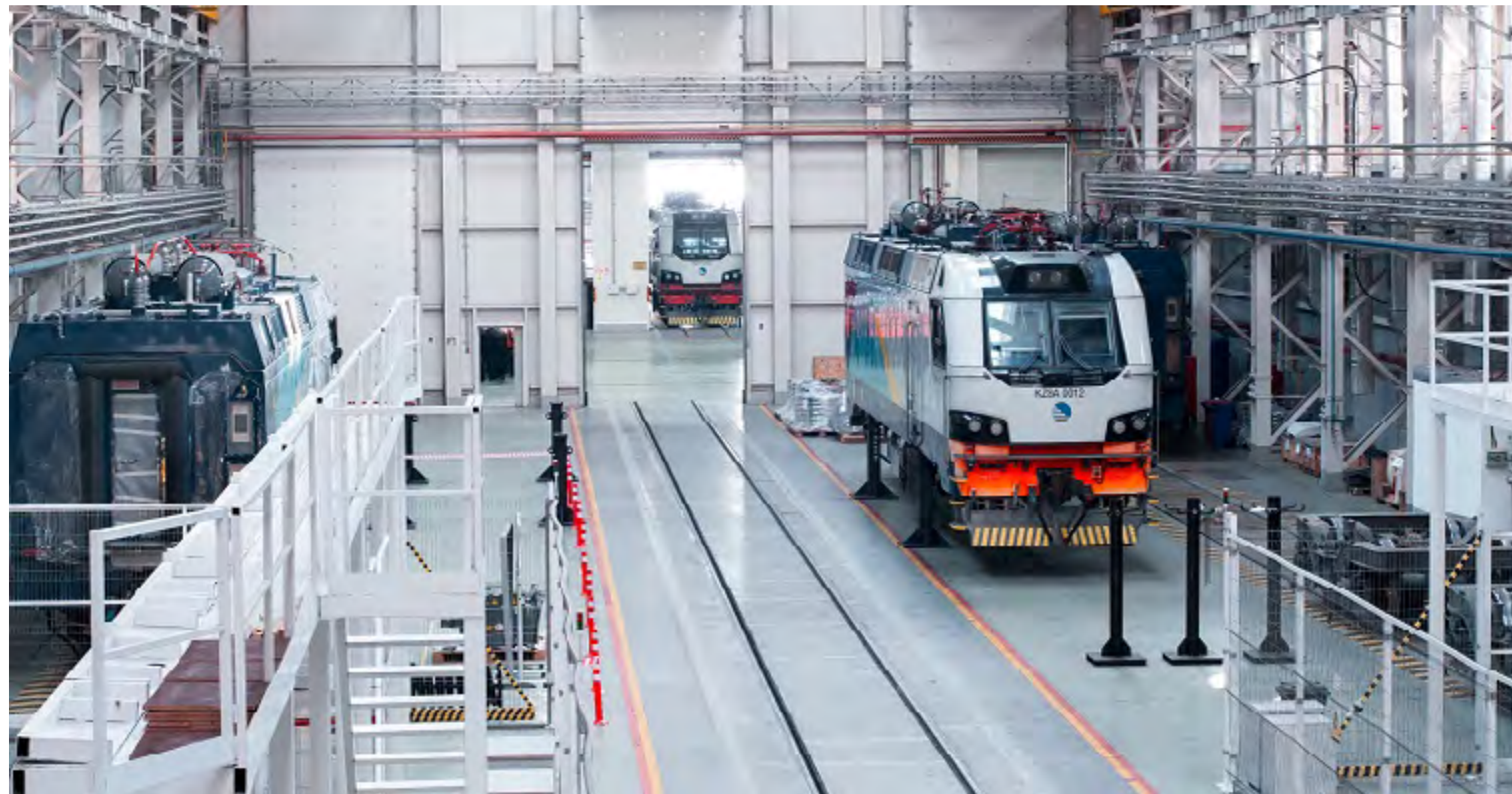
With 16,000 km of track, the Kazakh railway network is the world's third biggest network using the 1,520 mm track gauge and represents a substantial market for maintenance activities.
