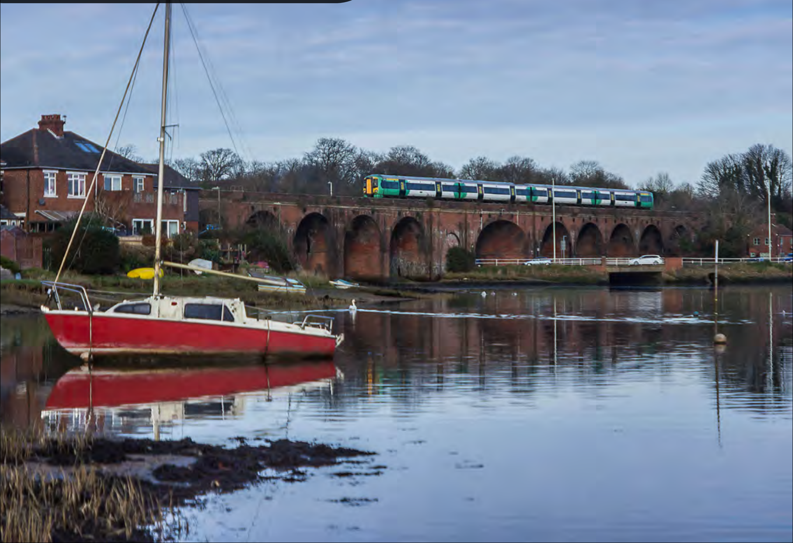
On January 16th, a Southern Class 377 EMU working the 11:47 London Victoria to Southampton Central via the Mid-Sussex line, crosses the Wallington river viaduct on the approach to Fareham. Stewart Smith
