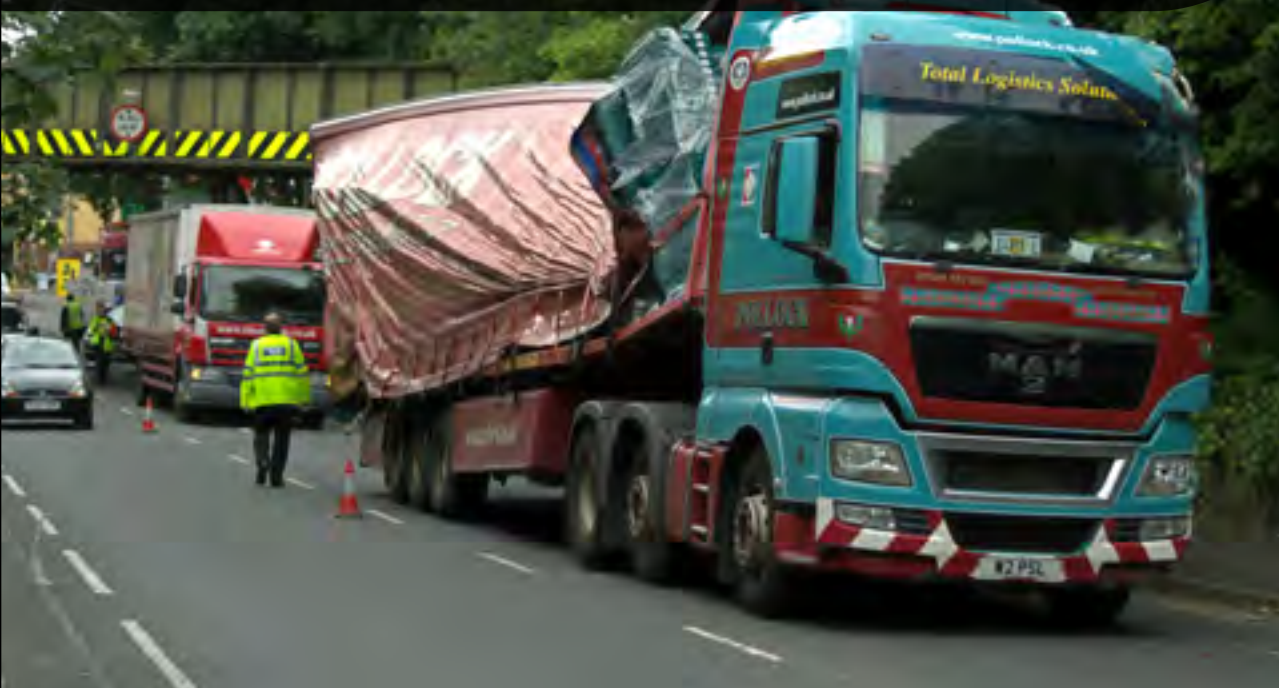
The aftermath of a Bridge Strike at Ewood, Blackburn is seen on August 5th. The driver clearly forgetting that big wagons don't fit under small bridges. Dave Felton
