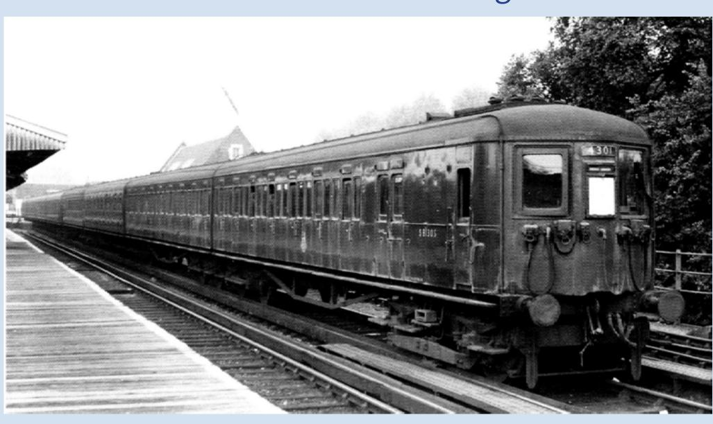
The Southern Railway obtained much of its stock for suburban electrification in the 1920s and 1930s by converting pre-grouping steam-hauled coaches. However the SR built two batches of new suburban electric stock in 1925 for the Eastern section and for the Guildford via Cobham line. The latter, seen here, followed previous LSWR electric stock by having a vee-nose instead of the usual flat front.
