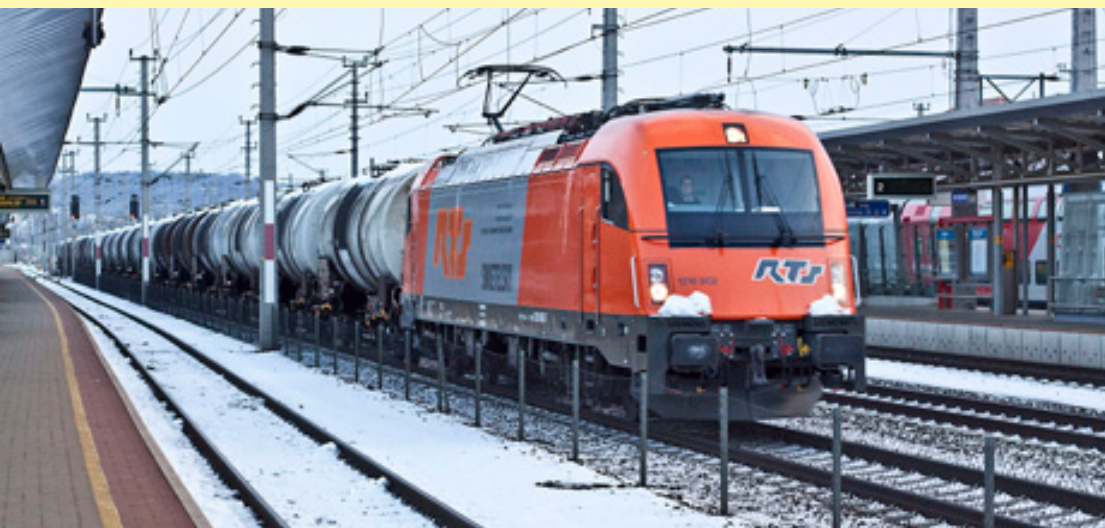
Top: A snow covered loco from the Mariazellerbahn line is pictured arriving at St. Pölten during a snow storm on 17th February. Class47
